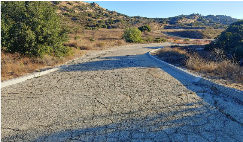
Figure 8. LOX Access Road Curb Extension
