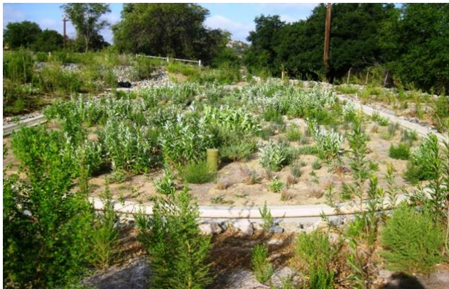
2013: Lower Parking Lot Sedimentation Basin and Biofilter
