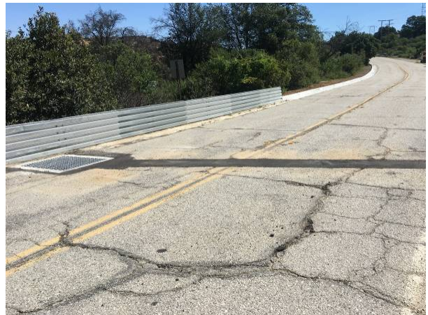
2017: Roadway Diversion to CM-3
