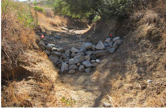
2012: Northern Drainage Restoration Measures
