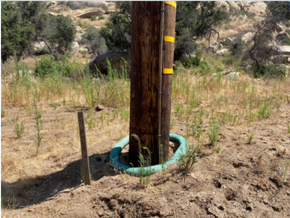
Figure 11. Media wattle installed around pole in Southern Buffer Zone
