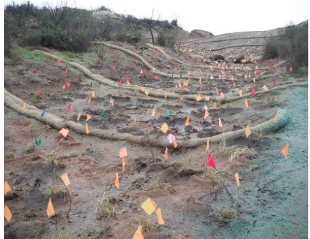
2010: Outfall 008 Watershed ISRA Excavations
