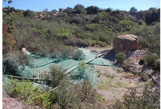
2012: CM-9 Additional Improvements (Perforated Pipe and Rip Rap Berm)
