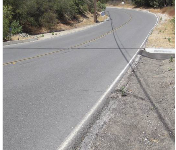
2017: Roadway Diversion to CM-1
