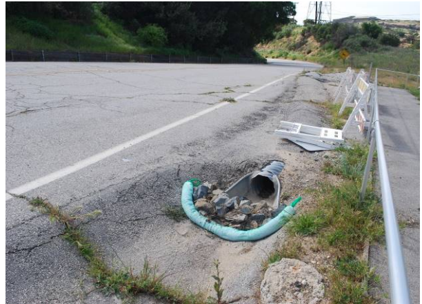
2017: Administration Area Weighted Wattle and Riprap at Culvert Inlet
