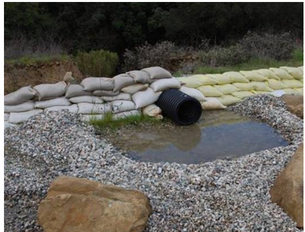
2013: LOX Sandbag Berms and Slope Drains
