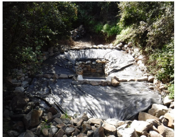
2020: Outfall 009 CM-3 Check Dams Added and Filter Media Reconstruction
