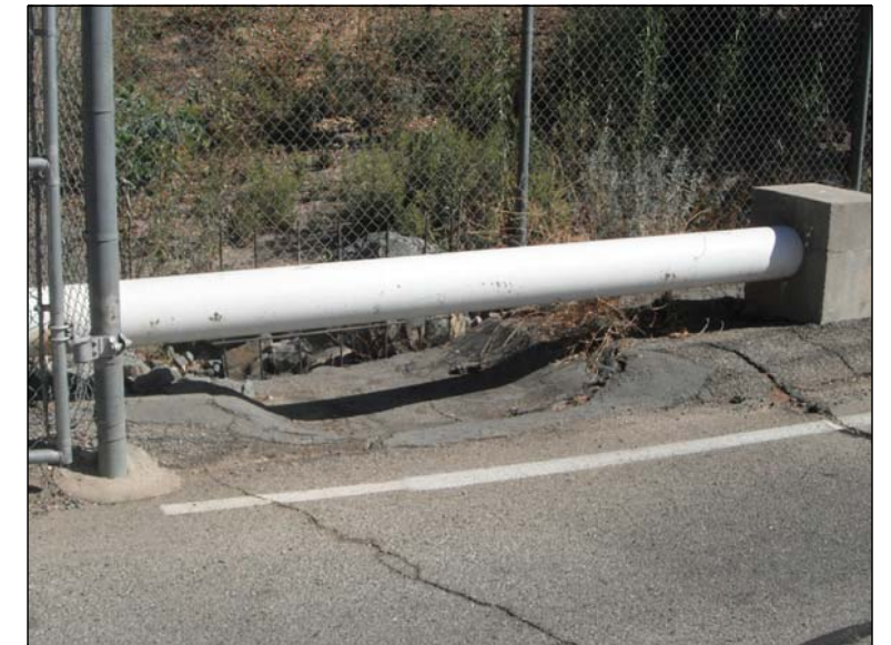
PHOTO #1: LOOKING SOUTHEAST AT EXISTING CURB CUT DRAINING TOWARDS EXISTING CHECK DAMS. THIS DESIGN IS RECOMMENDED FOR THE (3) 36" PROPOSED CURB CUTS.
