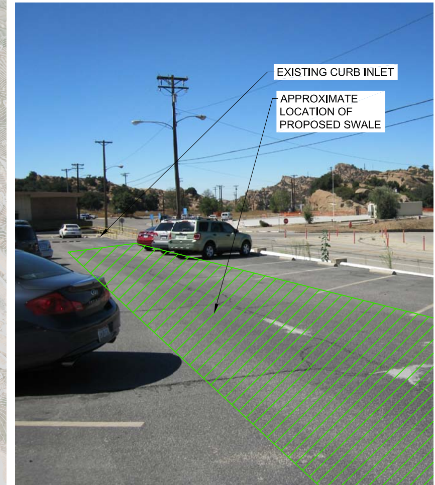
APPROXIMATE LOCATION OF PROPOSED VEGETATED SWALE AND CONNECTION TO EXISTING CURB INLET
