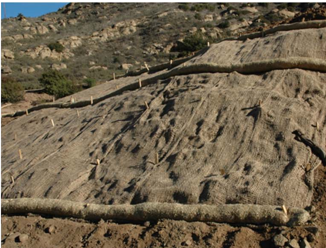
Erosion and sediment controls
