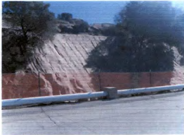
Jute matting installed on the slope in the B1-2 ISRA area.
