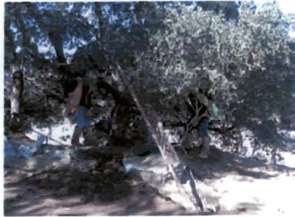
Backfilling around oak trees using hand tools.
