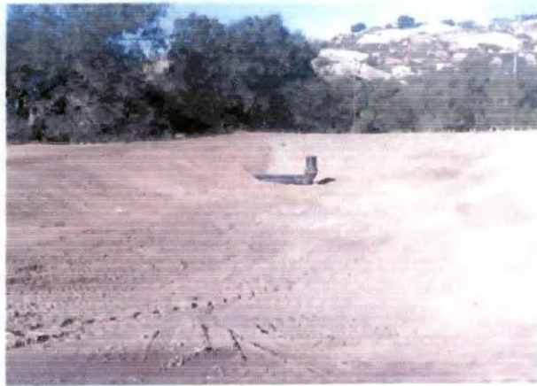
Temporary sediment control BMP (retention basin and discharge pipe) in the B1-2 ISRA area.
