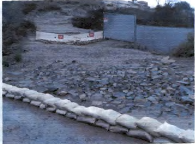
Restoration of access road to B1-1 ISRA areas.
