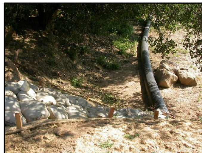
VIEW 3 LOOKING SOUTH
