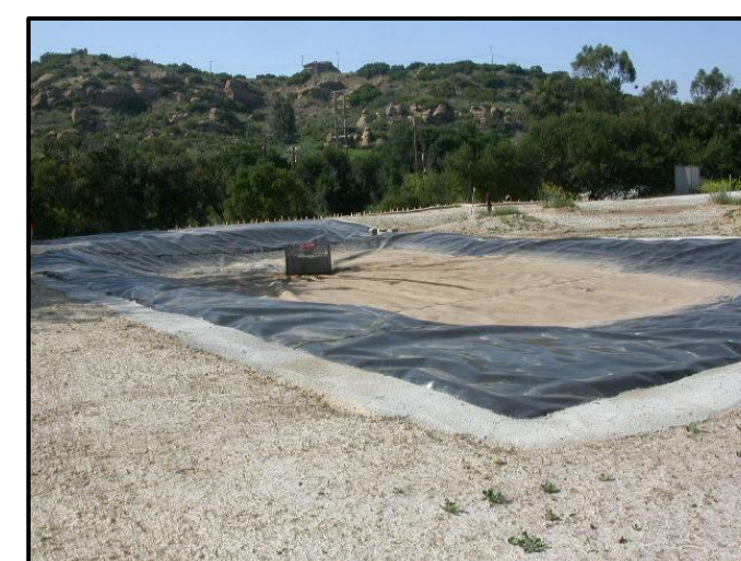
VIEW 4 LOOKING NORTH
