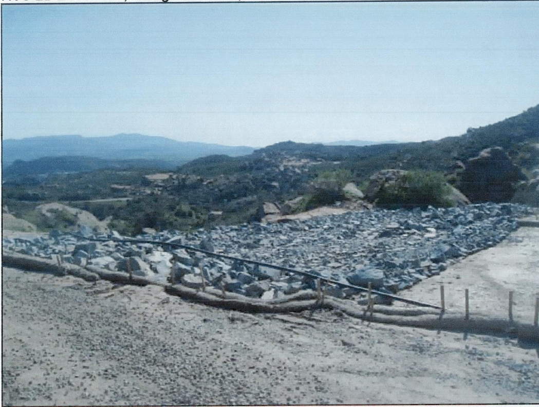
HVS-2B-2 rock crib, facing west, 2/17/2010:
