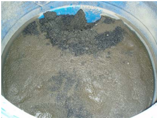
Clogged Activated Carbon (8/24/06)
