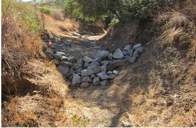
2012: Northern Drainage Restoration Measures
