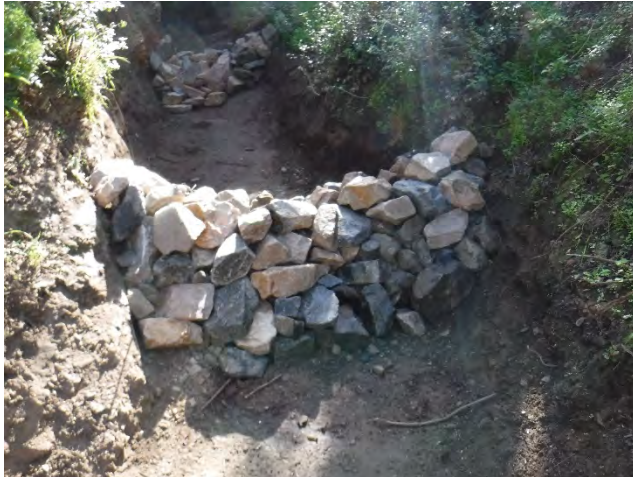
2020: Outfall 009 CM-3 Check Dams Added and Media Filter Reconstruction
