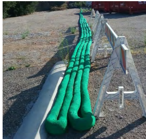
2019: Mulch Sack Curb Extension in Lower Parking Lot
