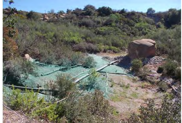
2012: CM-9 Additional Improvements (Perforated Pipe, Extended Sedimentation Area and Rip Rap Berm)
