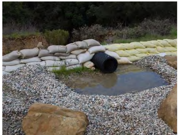
2013: LOX Sandbag Berms and Slope Drains
