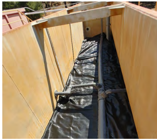
2021: Outfall 009 ELV Treatment BMP Media Filter Reconstruction
