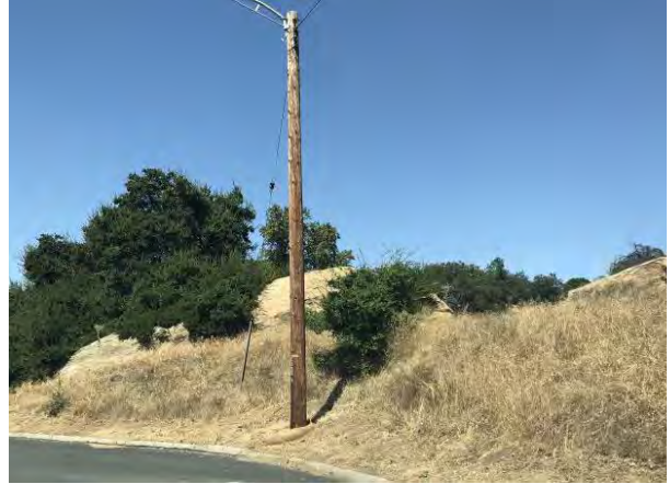
2017: Wattles around Poles along Roads
