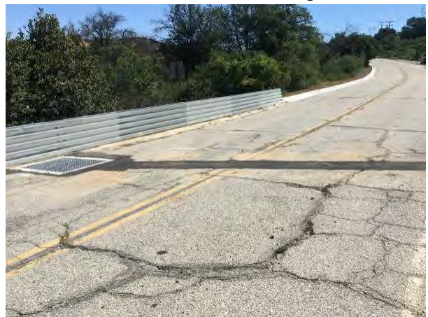
2017: Roadway Diversion to CM-3
