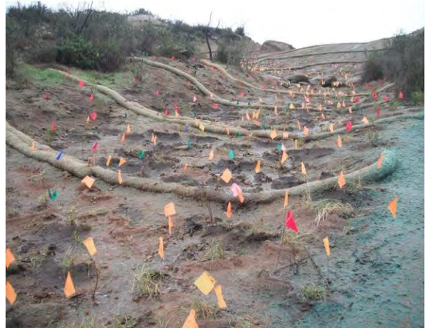
2010: Outfall 008 Watershed ISRA Excavations
