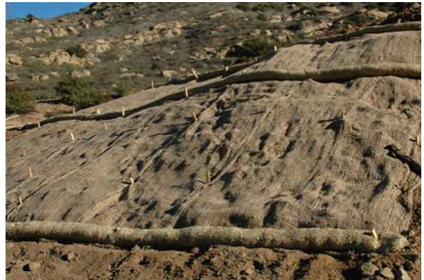
2013: Outfall 009 Watershed ISRA Excavations
