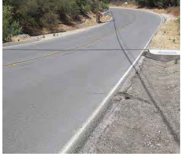
2017: Roadway Diversion to CM-1
