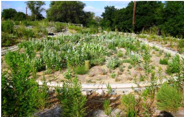
2013: Lower Parking Lot Sedimentation Basin and Biofilter
