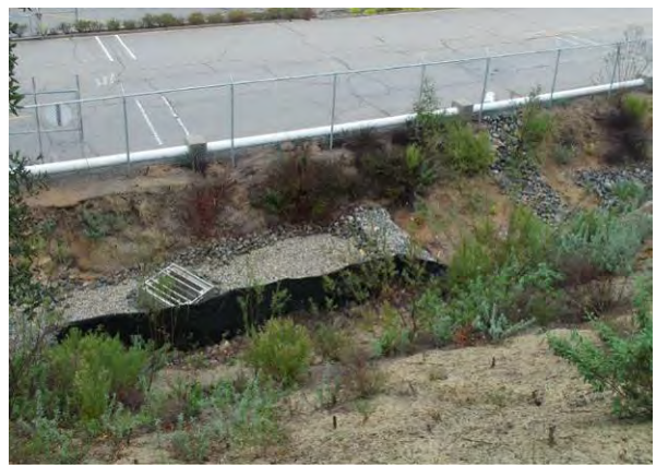
2012: B-1 Sedimentation Basin and Media Filter
