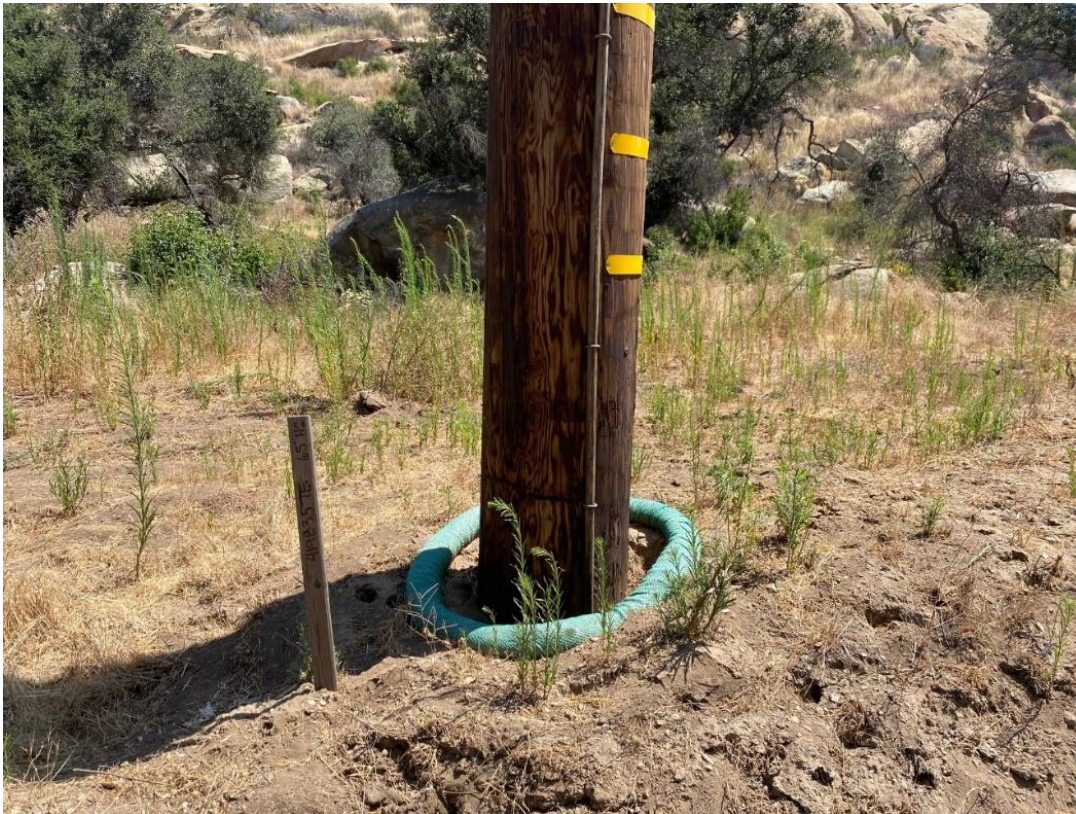
Wattles added to approximately 115 Poles
